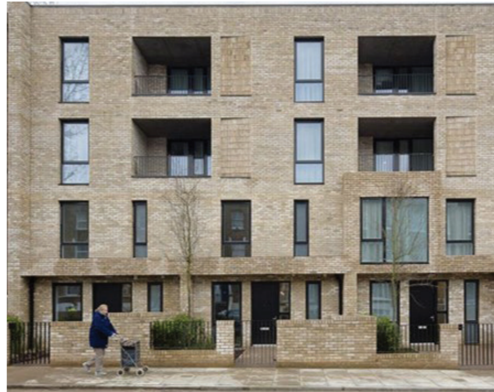
TYPICAL BRICK EXEMPLAR CLADDING
